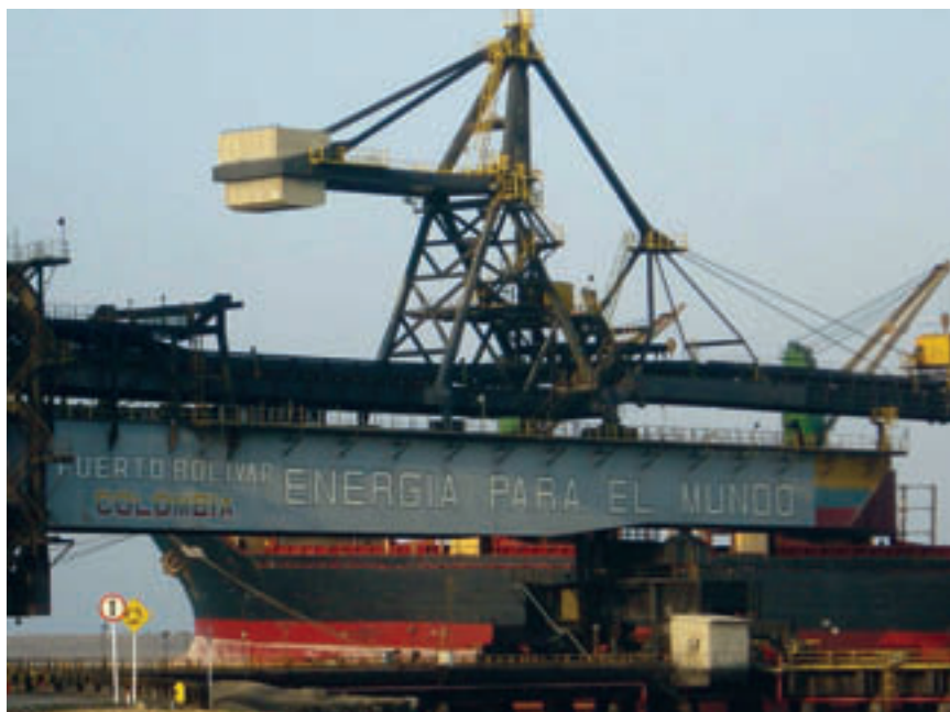
↑ Coal terminal at the Puerto Bolivar in Colombia
